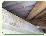
When we are called to an owl removal, it's because the birds have nested in the roof space of a home, school or office building. Gaps larger than 4" between the walls and roof can be sealed with wire mesh, foam or wood to keep the owls out. This makes sense since
